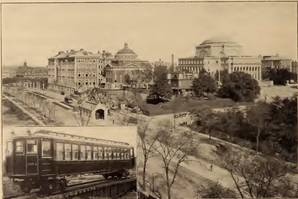
UNIVERSITY STATION BROADWAY AND 116TH ST. View North showing Columbia University. Vault lights over Subway; ventilation shaft inclosed in railing, parkway over subway, surface cars, etc. Station decorated appropriate to University. Subway steel car at left.
